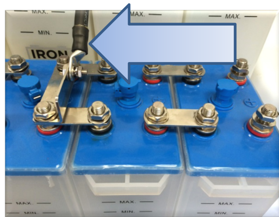
2 Batteries Bypassed
